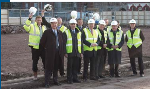
Hats off to the team for the start on site of Liverpool's most prestigious residential development, 'L1'. Our CMPB staff are shown here with the client, Windsor Developments (Liverpool) Ltd and representatives from the main contractor, Laing O'Rourke and from architects, Downs Variava.
